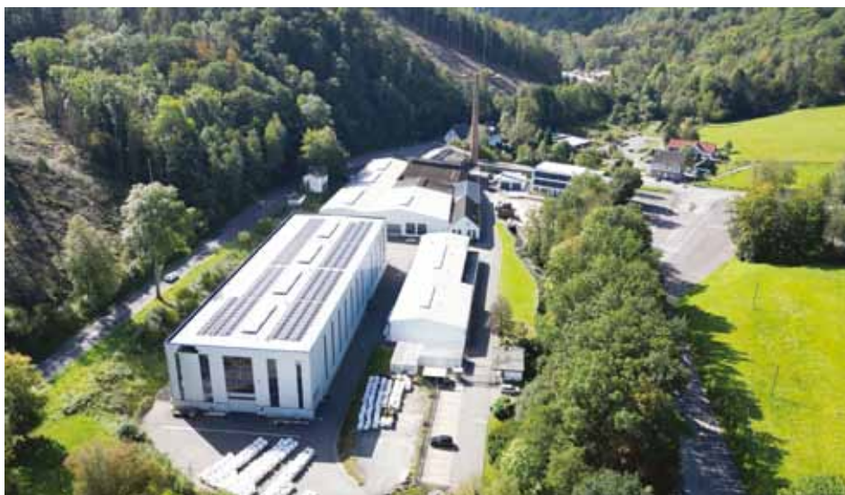
Substantial investments are planned to continue upgrading the Kind facility in Kaiserau, Germany.
