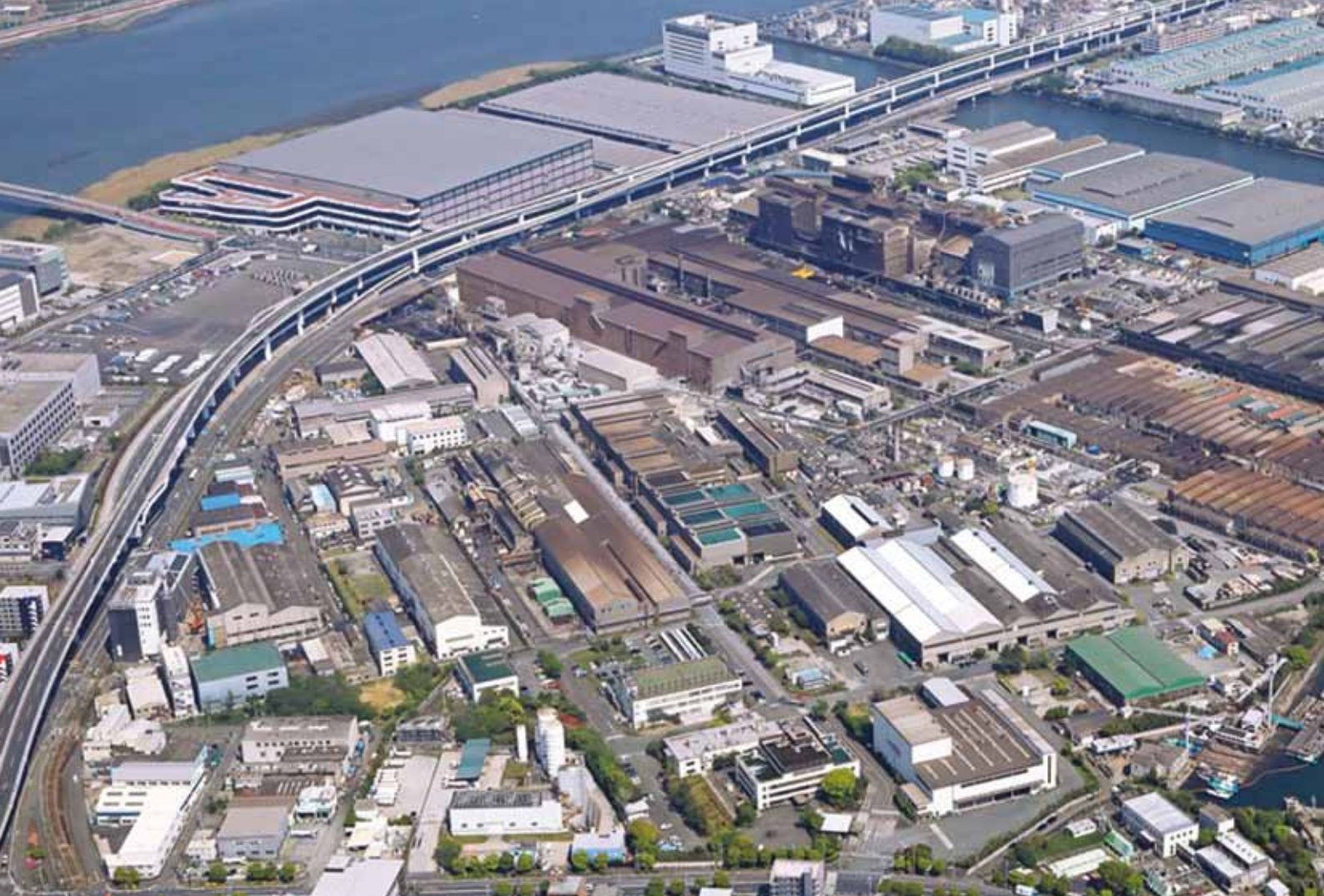
Nippon Yakin Kogyo's flagship production facility in Kawasaki, Japan.
