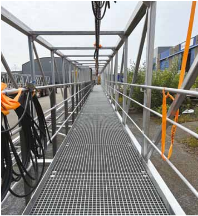
The use of lean duplex instead of carbon steel resulted in a considerably lighter structure while almost eliminating the need for maintenance.
