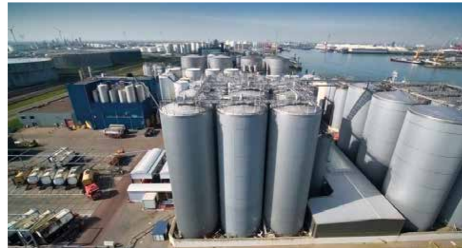
Outokumpu inspected tanks which have been in service for years to obtain documented information available about the service performance of actual structures.
