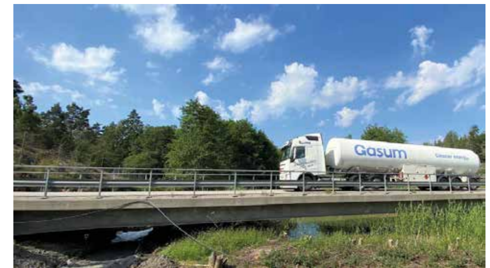
The high strength, minimal weight and long life of duplex of the Nynäshamn bridge fits with increasing focus on reducing the lifetime carbon footprint of infrastructure.
