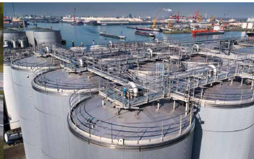
In the ATM tanks inspected near Rotterdam, Forta LDX 2101 showed good resistance to atmospheric corrosion after eight and twelve years in the service environments.
