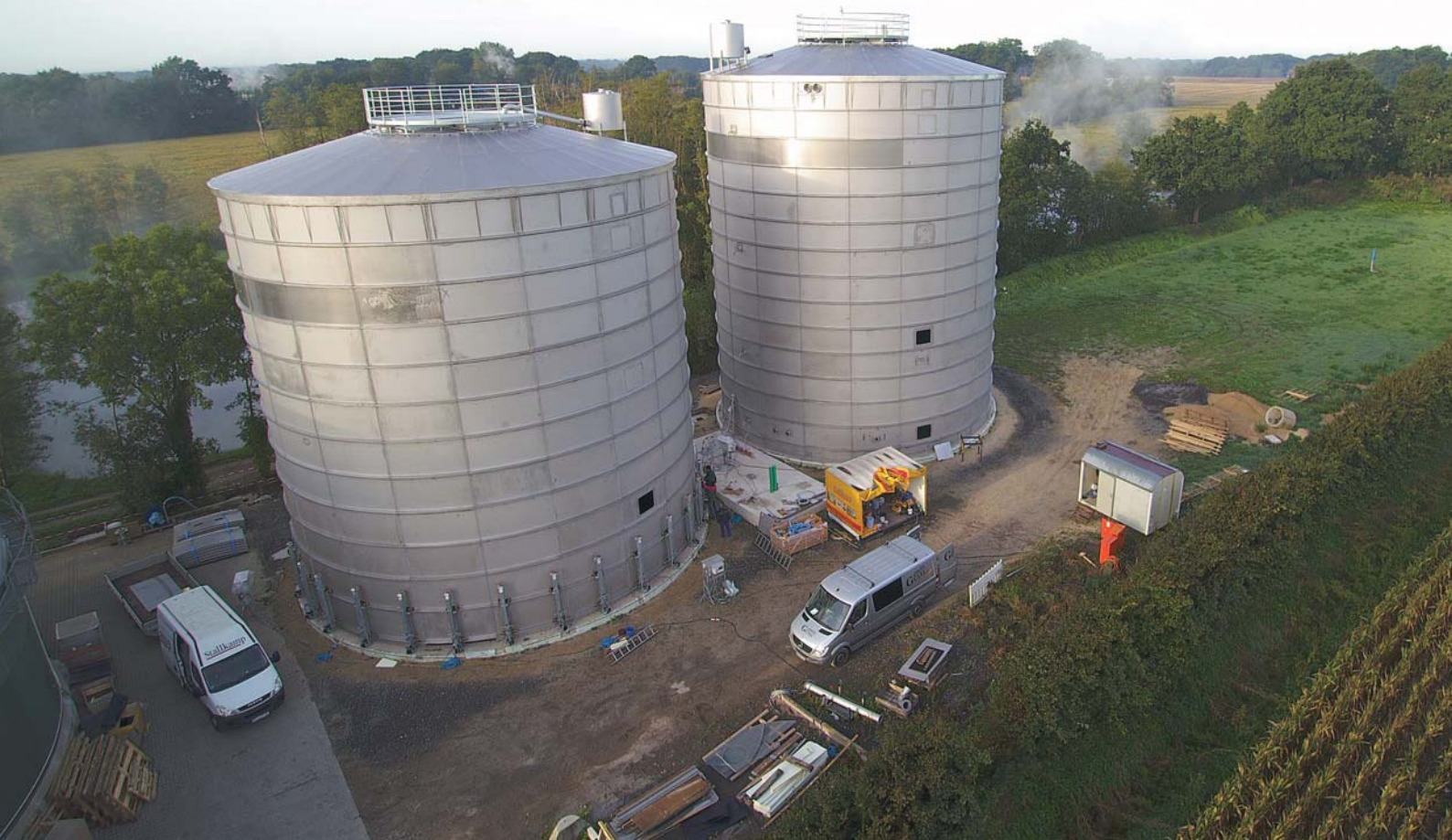
Continuously stirred tank reactor in stainless steel during construction.
