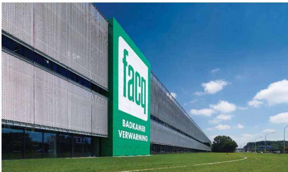
The façade's outer metallic surface is almost opaque, making it an ideal sunshade. Source: Haver & Boecker.
