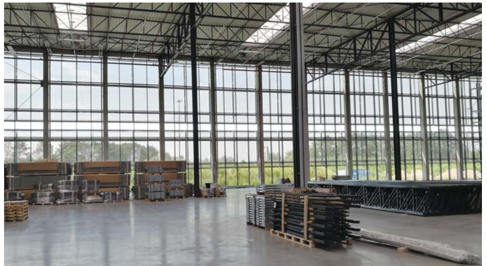
View from inside FACQ building, demonstrating the near transparency of the mesh when looking out. Source: Haver & Boecker.
