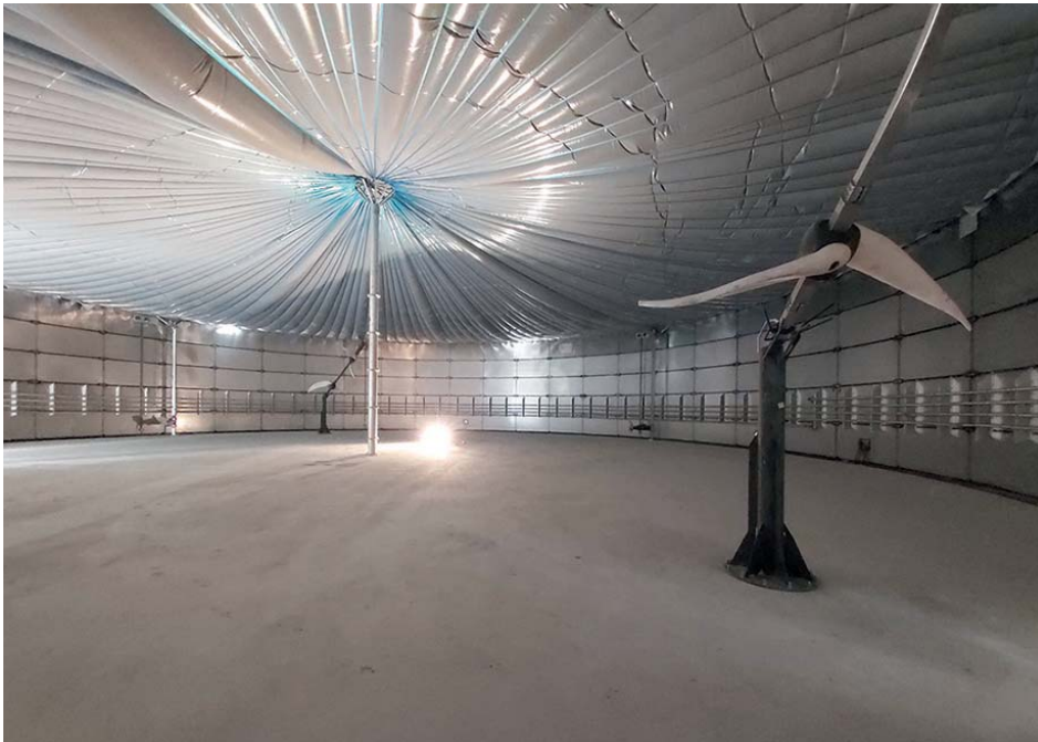
Currently, three fattening houses are being built in addition to the existing piglet production sites. In this way, some 40,000 t of pig manure are available as input material for the stainless-steel digester, which has a capacity of 4903 m 3 .
