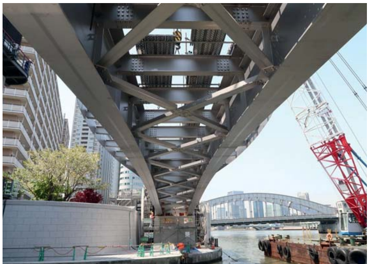
NSSC 2120 duplex is increasingly specified for public infrastructure, such as the bridge connecting esplanades along the Sumida River in Tokyo.
