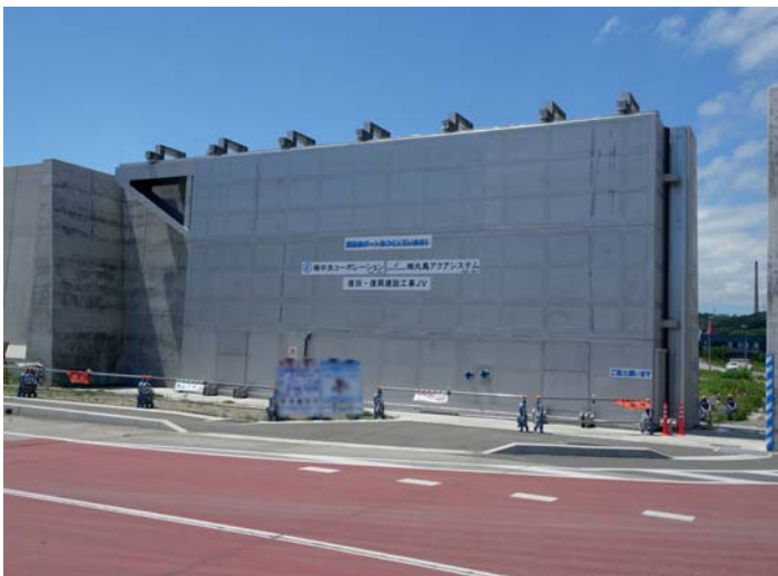
A land lock for flood/tsunami protection constructed from NSSC 2120 duplex.
