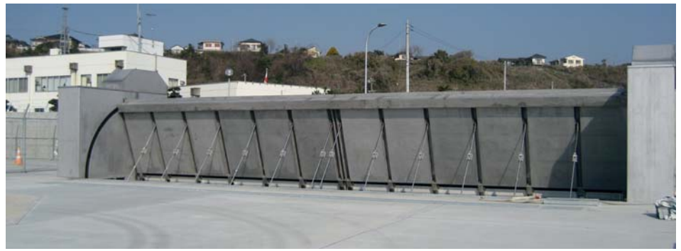
NSSC 2120® stainless steel Flap-Gate type Seawall against flood disaster won the Bronze Award in the category of New Technology and New Development during the 22nd Annual Conference of International Stainless Steel Forum (ISSF).
