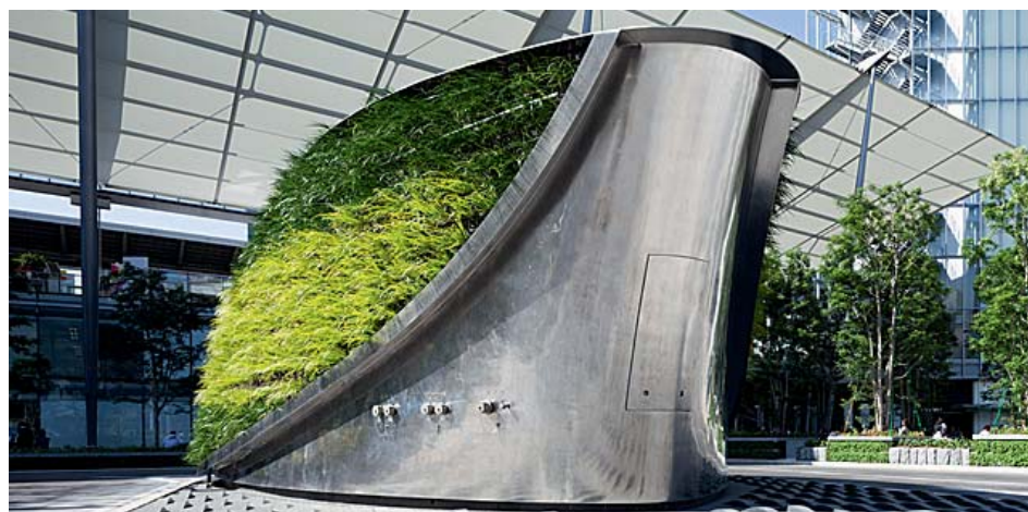
The duplex plates made by NSSC were applied for the ventilation tower at the Yaesu Central Entrance of Tokyo Station.
