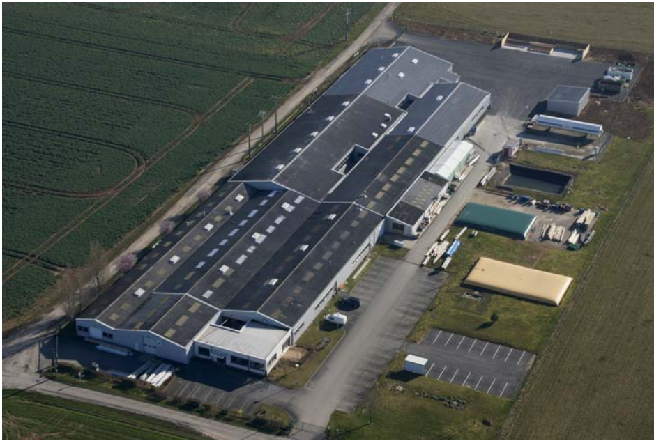
An aerial view of the SOTEP tubes plant in Issoudun, France.
