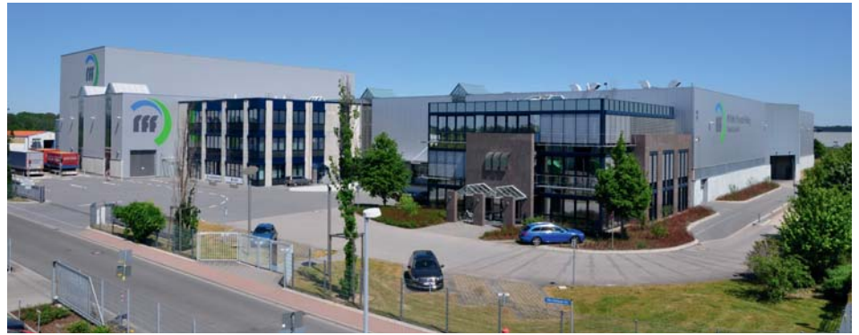
The inauguration of the new pipe cassette storage took place in Beucha / Leipzig In April 2009.
