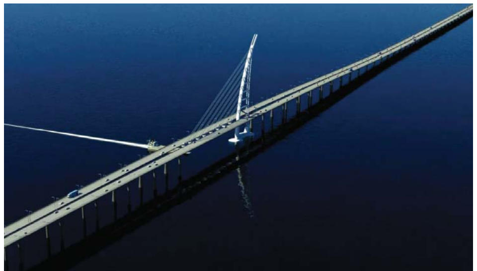
The Sheikh Jaber al-Ahmad Al-Sabah Bridge in Kuwait: 1,600 metric tons of stainless steel rebar Forta DX 2304 was used for the 36 km long causeway project. The bridge is expected to be in service by the end of 2018.
