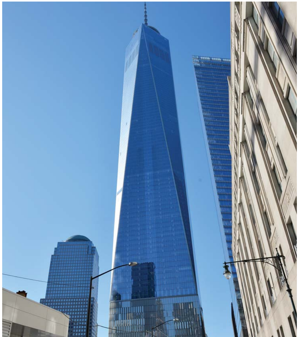
The One World Trade Center is the architectural landmark in Lower Manhattan, NY, USA. Two hundred tons of Laser-finished cladding, made in Dillenburg, Germany, was delivered to the construction site. Architects like stainless steels 'honest' and 'pure' qualities, as well as its noble appearance.
