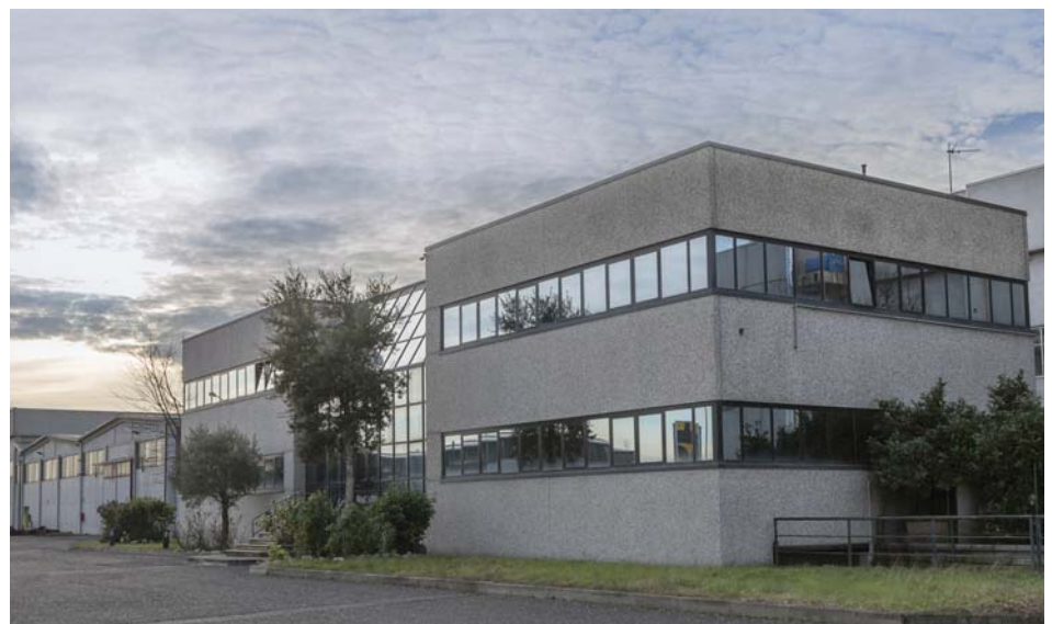
Petrol Raccord plant in Calendasco (Piacenza, Italy), home to the Group's latest addition.
