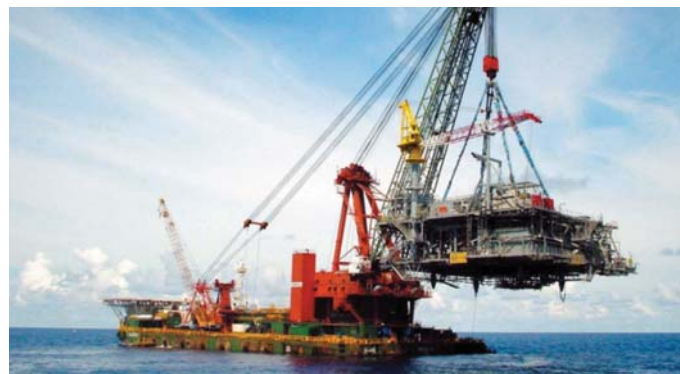
DP3W, 25Cr super duplex stainless steel is widely used for offshore piping systems as well as umbilical tubes.
