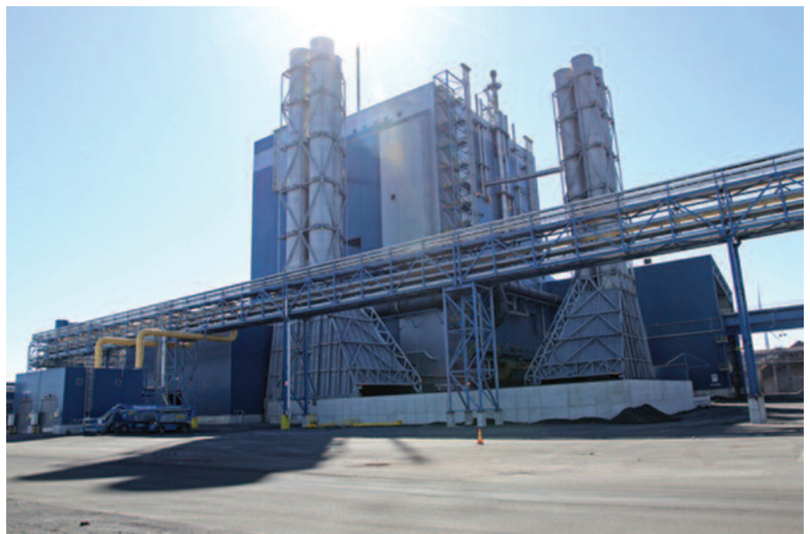
The new ferrochrome works in Tornio, Finland, June 2013.
