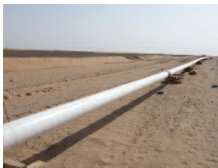
API 5L CRA welded line pipe LC65-2205 supplied by Jiuli at a PDO project site in Oman.
