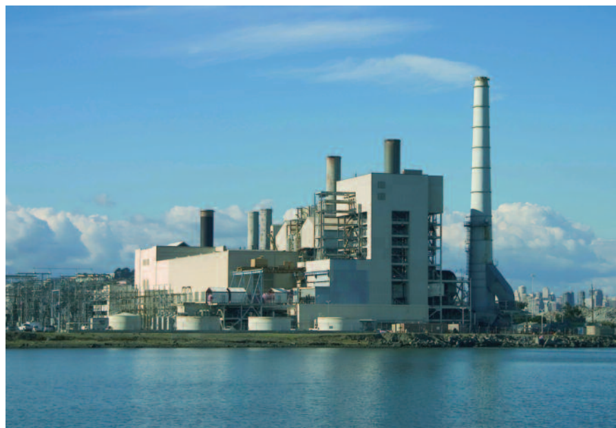
The power generation industry is developing new, highly efficient technologies and plants with a growing need for seamless stainless tubes.
