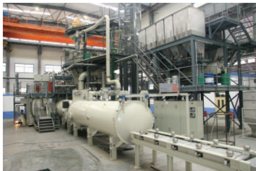
Electron beam cold hearth melting furnace.
