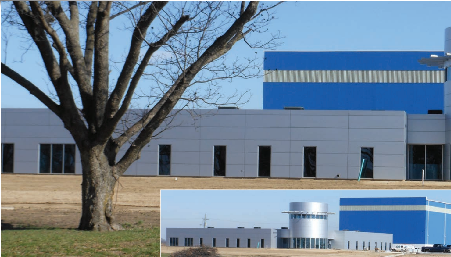
The Schulz Group of Companies' state-of-the-art seamless pipe mill in Tunica, Mississippi, USA as photographed in November 2011. In less than two years the 130 million US-dollar investment for subsidiary Schulz Xtruded Products has been constructed and the first pipes have already been manufactured.
