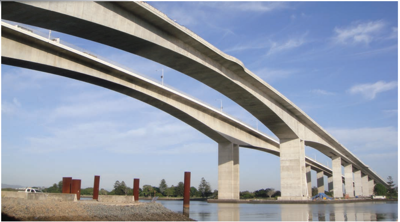
Outokumpu Duplex LDX 2101® stainless steel reinforcement bars (rebar) were used in critical sections susceptible to corrosion, in two columns at the bases of the breakwaters on the Brisbane Gateway Bridge, Australia. Photo courtesy of Leighton Abigroup Joint Venture ABN.
