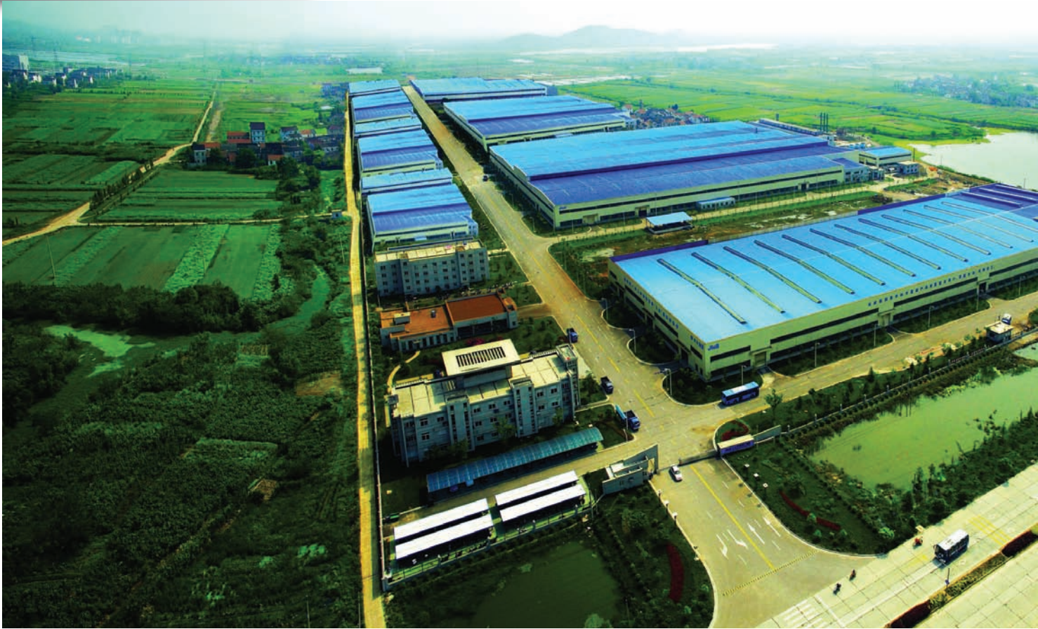
Jiuli's new expanded industry park for seamless pipes/tubes production.
