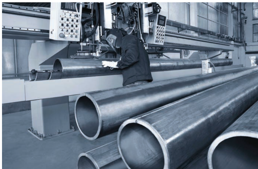
One of WPI's qualified welders at work.
