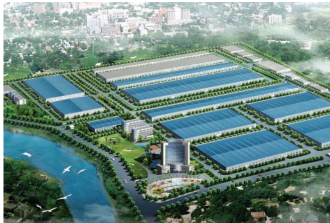
Bird's eye view of Baoti Industrial Zone
