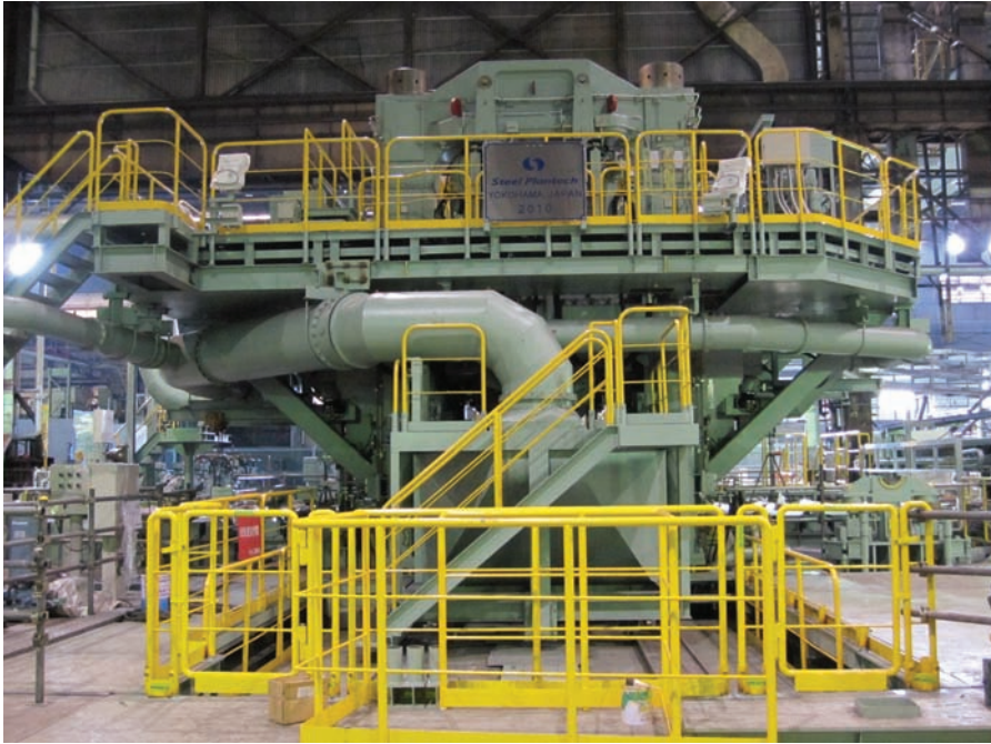
New cold-plate leveller almost ready for operation
