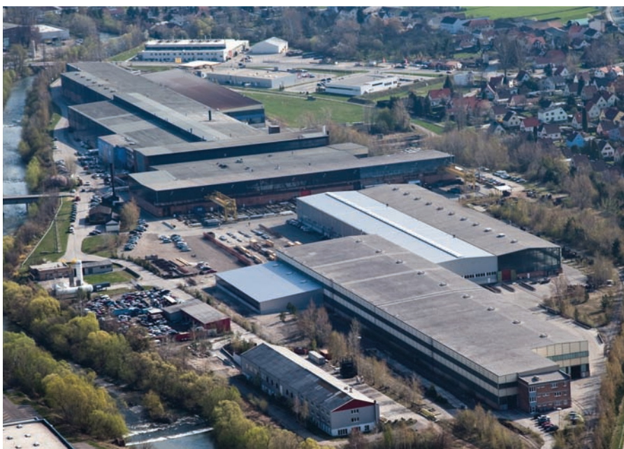
Schoeller Bleckmann Edelstahlrohr hosts over 50 million EUR of new investment.
