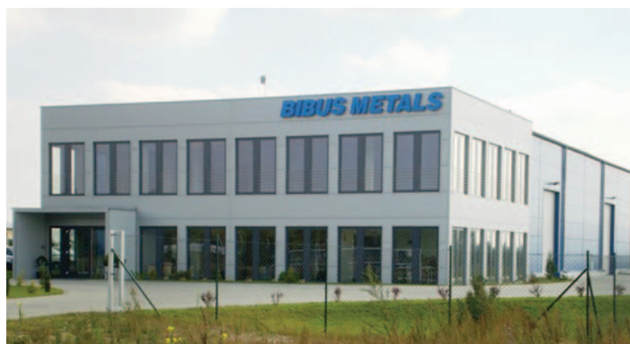
The BIBUS METALS Poland offices and warehouse.
