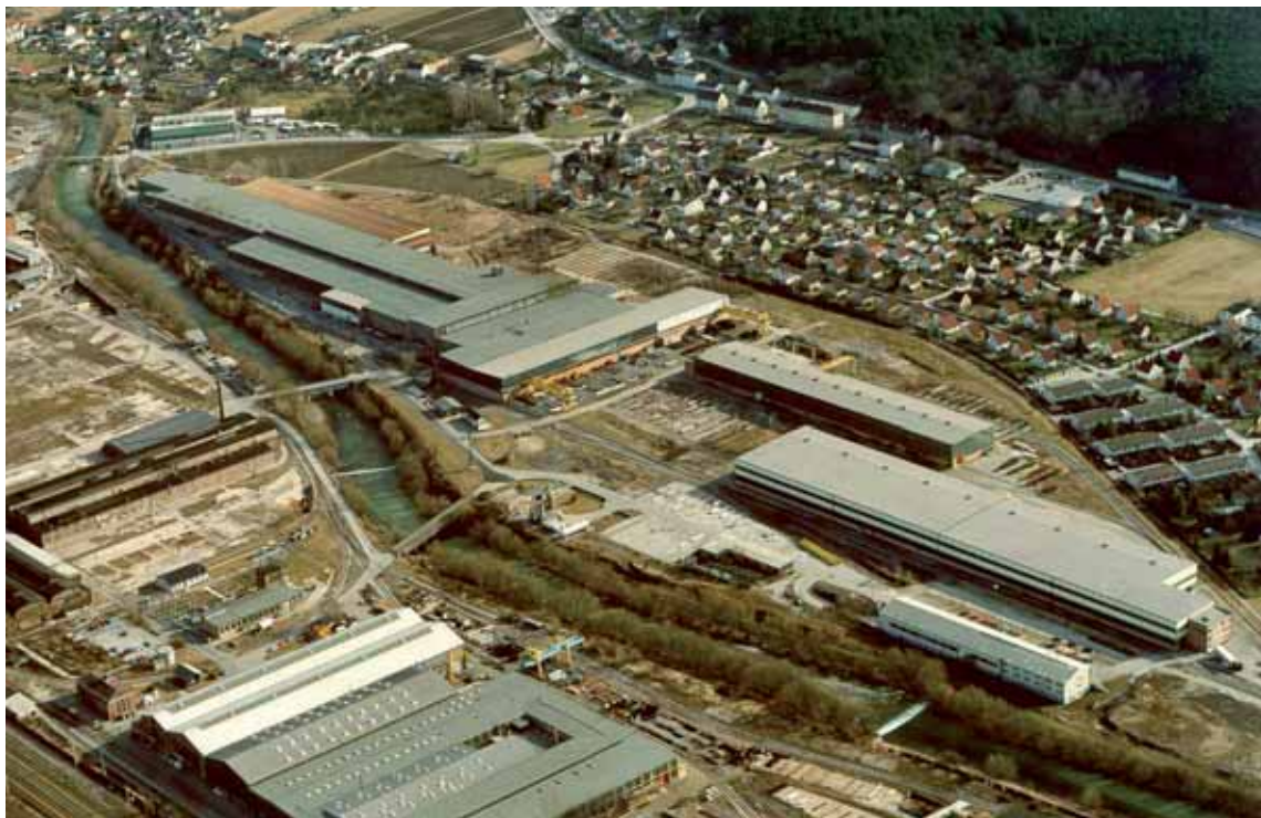
The integration between Austrian and Spanish facilities is better than ever.
