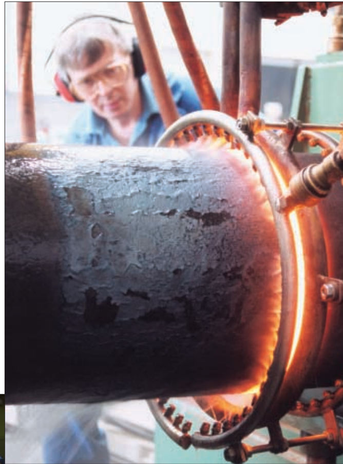
Induction Bending of 14" weld overlay clad pipe.
