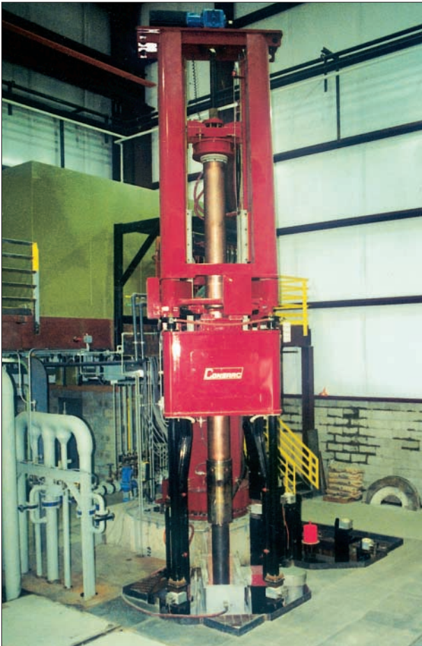
The new remelt installation at Electralloy features two of the largest furnaces operating in North America. The electroslag remelt unit (shown above) and the vacuum arc remelt unit can both process rounds up to 40 inches diameter.
