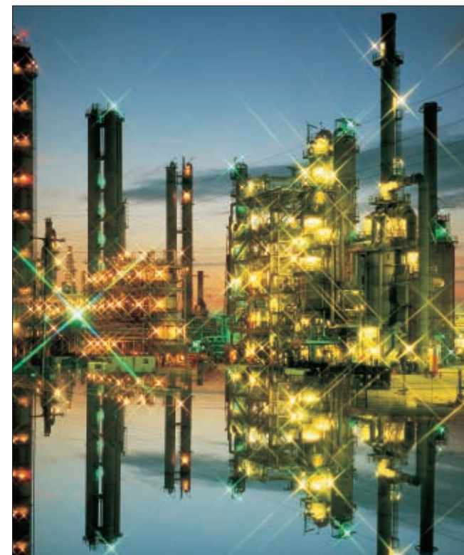
One of the most important customers of Hempel's Germany based operation is the chemical industry.
