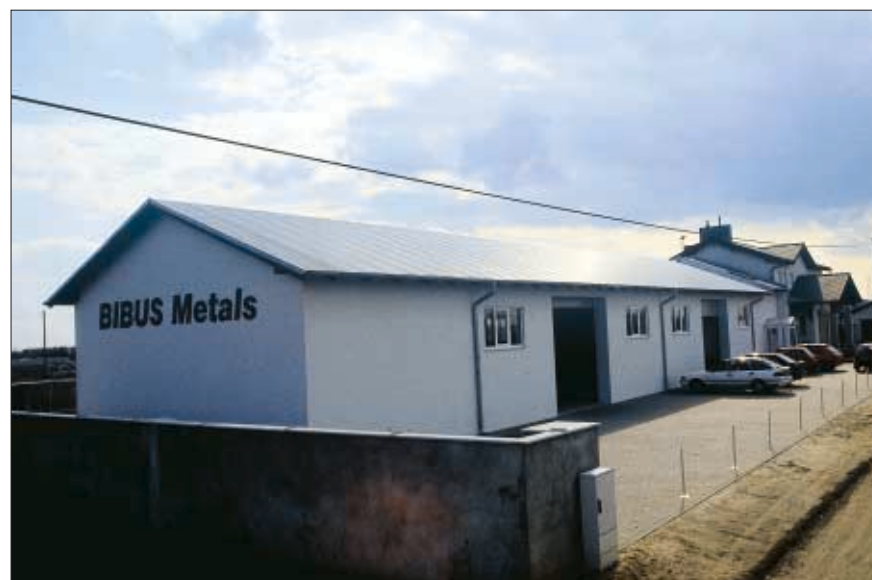
New warehouse in Poznan (Poland)
