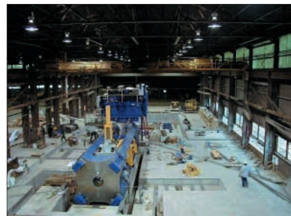
Installation of RTI's new extrusion press in Houston.
