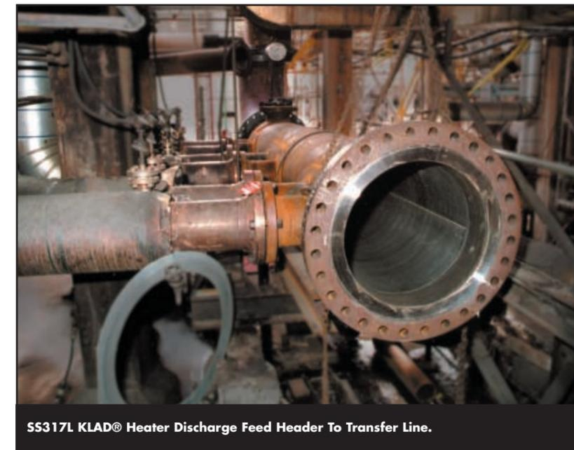
**SS317L KLAD® Heater Discharge Feed Header To Transfer Line.**
