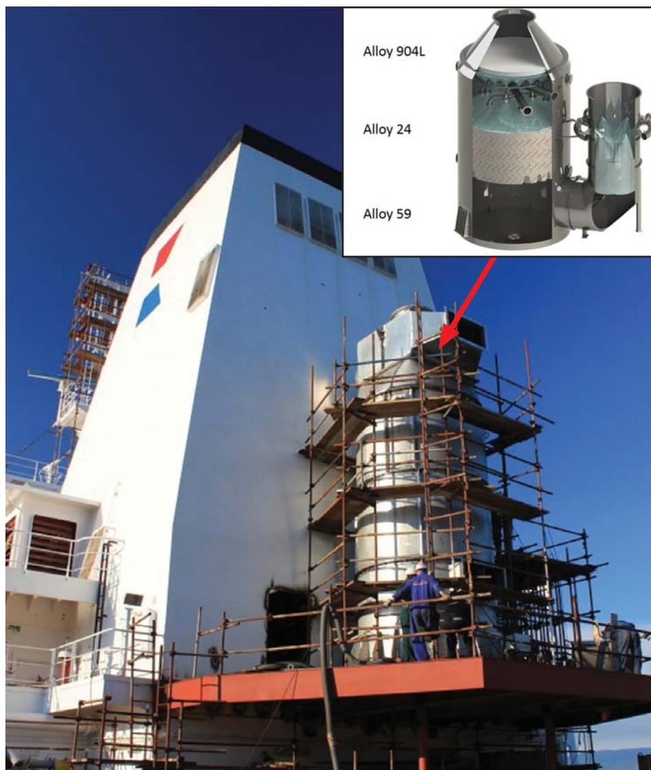
Hempel suppliers Alloy 24, 904L (1.4539) and Alloy 59 (2.4605) for scrubber technology designed in German and built in China. Pictures courtesy of Saacke GmbH
